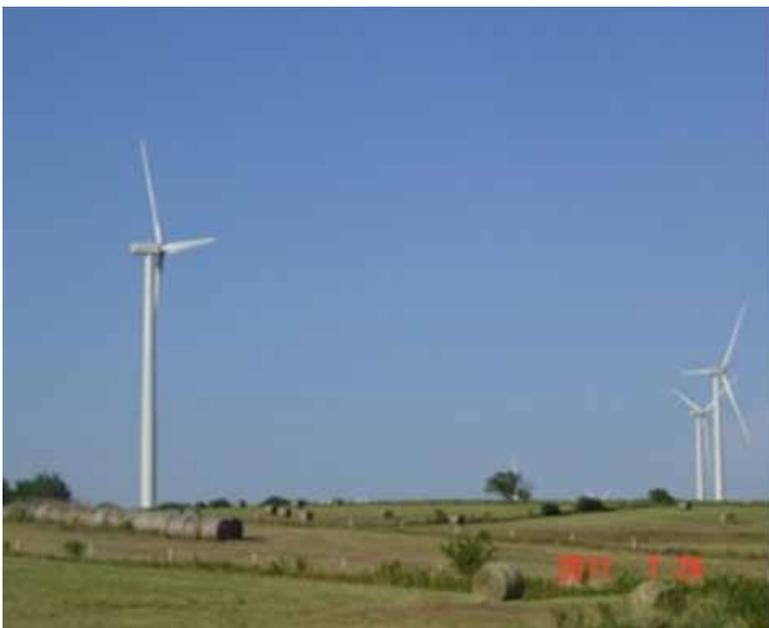
In practical terms, wind turbines share characteristics of both real and personal property. The turbine tower, constructed of steel sections that are bolted together, is attached permanently to a reinforced concrete foundation that is poured, beginning ten feet below grade. The turbine blades are typically made of composite material and attached to a nacelle atop the 350-foot towers. The nacelle, the size of a boxcar, houses the generator and other necessary mechanical apparatus.
